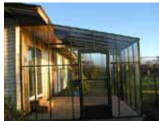
The attached greenhouse below has a four foot infill area to seal to the attaching wall.
